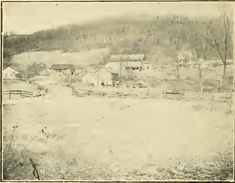
HOMESTEAD OF PETER J. FAUST NEAR SIGMUND, PA. The Site of the Old Hampton Furnace Property.
