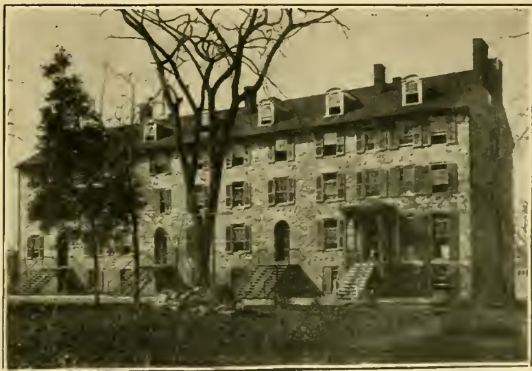
DICKINSON COLLEGE, CARLISLE, PA. EAST BUILDING.
